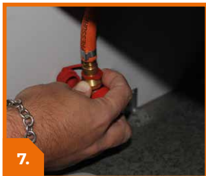
7. WITH GAS OFF PUSH DOWN ON BRASS NECK
